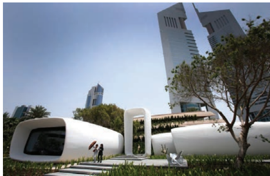
Dubai's 3-D printed office building.
